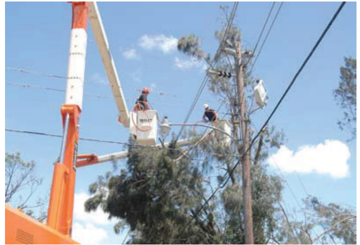
Figure 5. Only qualified line-clearance arborists can work on trees near power lines.
